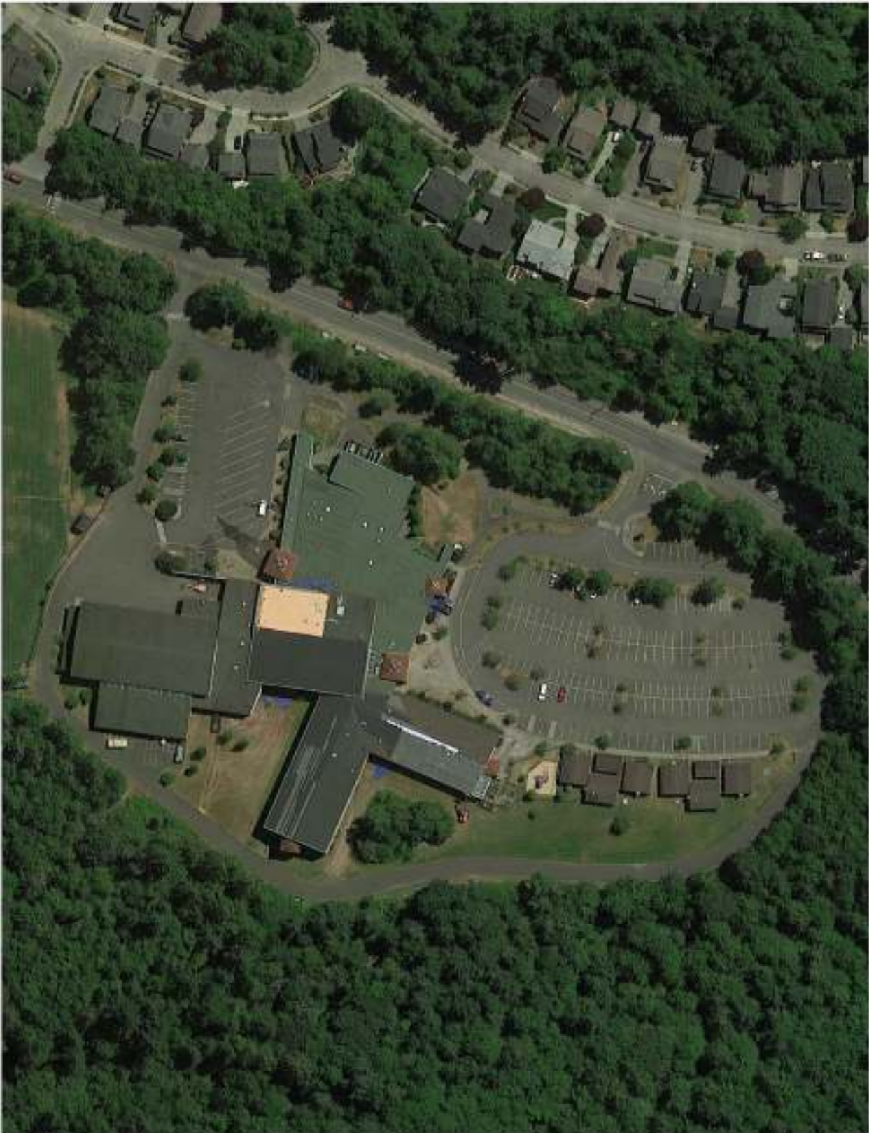
Woodward Middle School :: Existing Condition (98,516 gsf)
