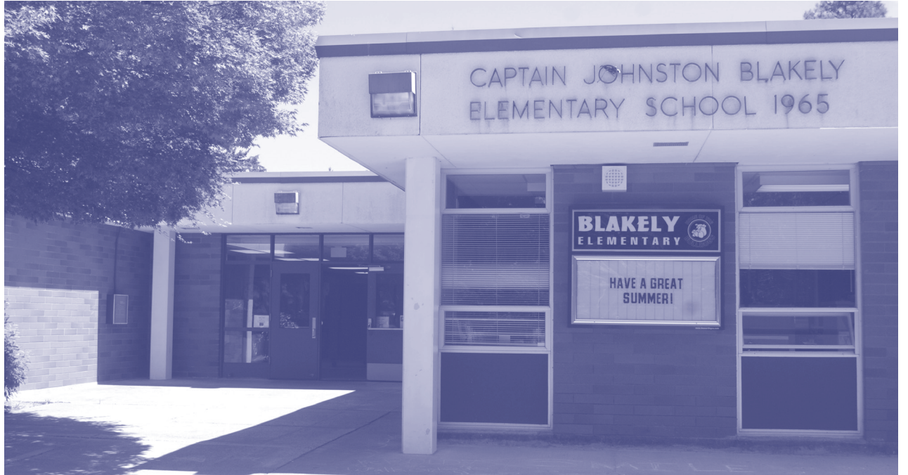
Blakely Elementary School is one of four district facilities with significant structural, mechanical, electrical and design deficiencies.
